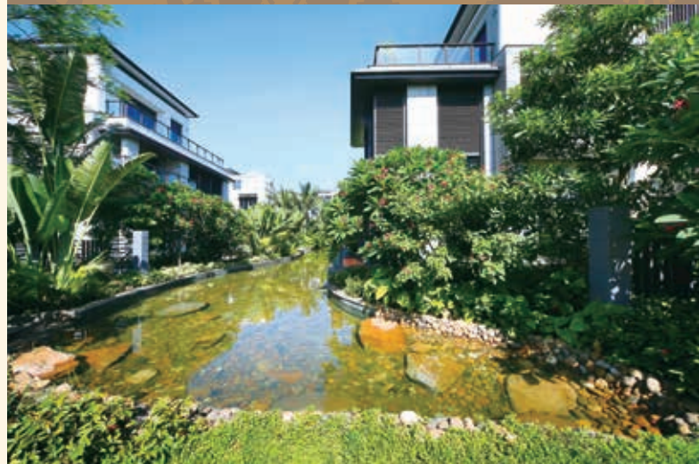
Haikou New World • Meilisha Project makes use of a seawater circulation system
