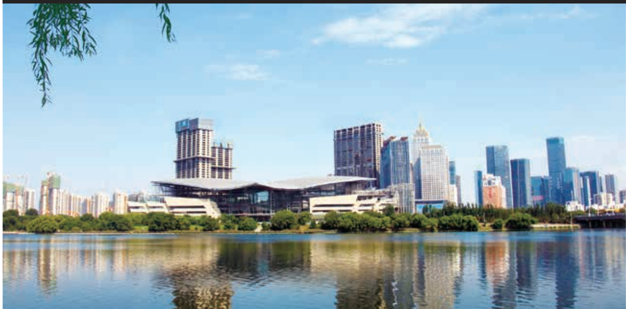
Shenyang New World Centre (under construction)
