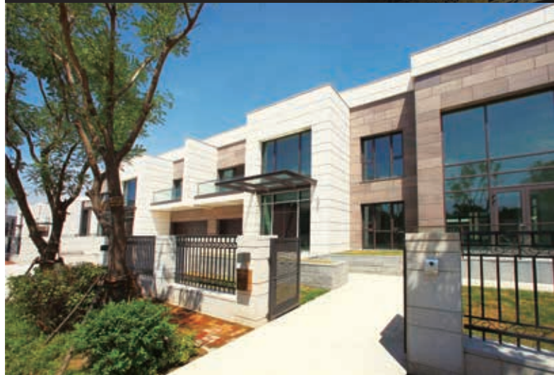
Shenyang New World Garden Phase II "New World • The Masterpiece Crescent"
